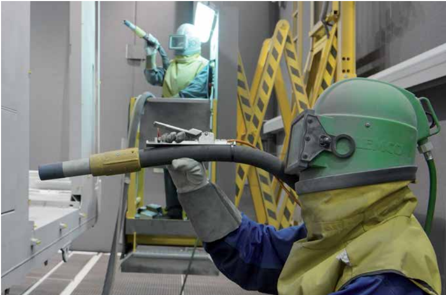
Blast room for rail vehicles, equipped with scissor-type lifting platforms
