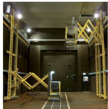
Blast room with scissor-type lifting platforms
